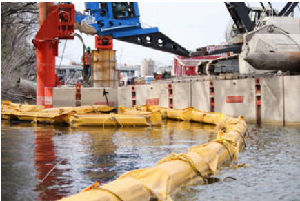
Construction on the Boardwalk Trail at Lady Bird Lake in March 2013.
