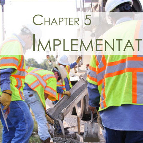
City of Austin Concrete & Asphalt Crew
